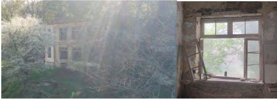
Figure 2. Sanatorium façade and recorder positioned on a room's windowsill photos by Christos Schoinas and Nicolas Remy (May, 2024)
