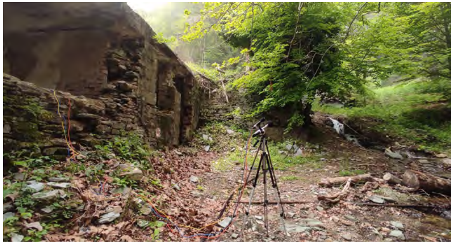
Figure 2a. From right to left, there is a view of the small river, the position of the microphones for the calibration setup, and the facade of the kitchen of the sanatorium. Sections 2b and 2c zoom in on the microphone setup
